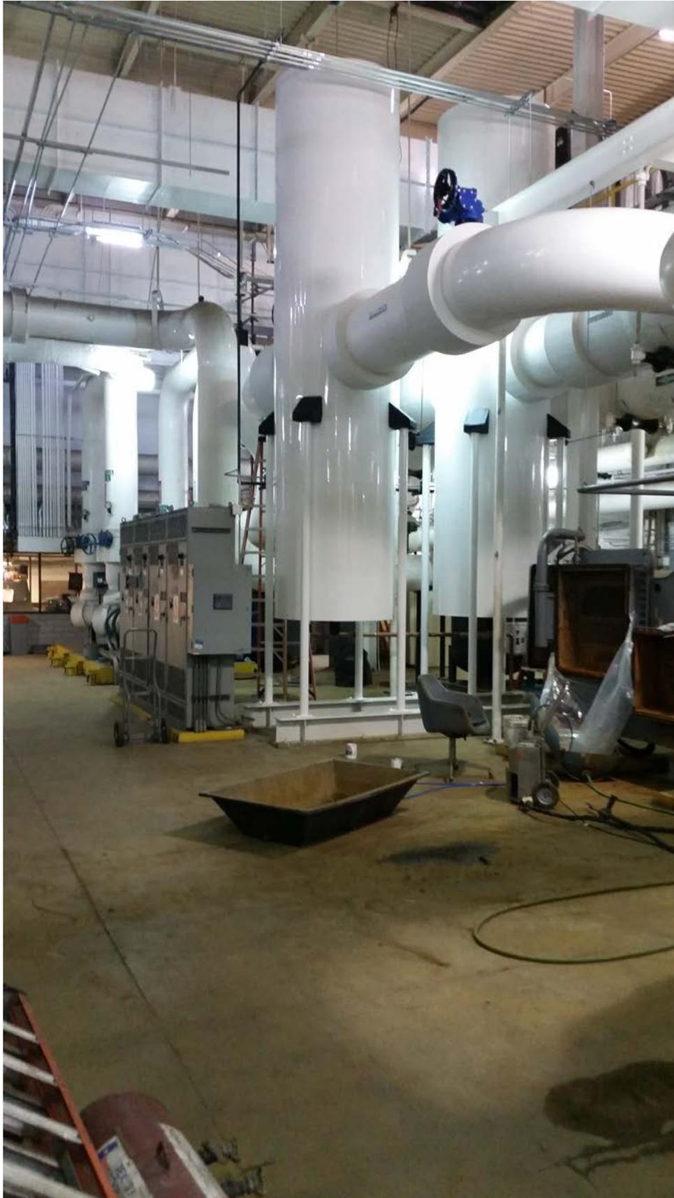
**Performance Contracting – Installed Coalescing Air Separators**
